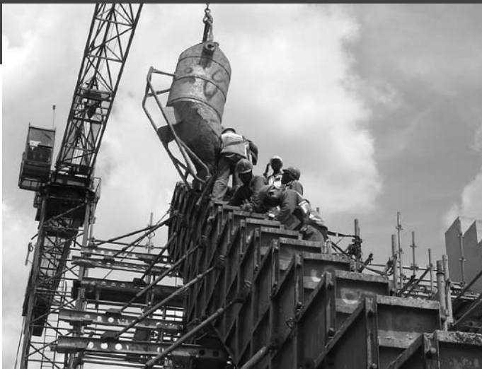
Picture: Workers preparing stadium pillars at Bhomebela Stadium, Nelspruit
